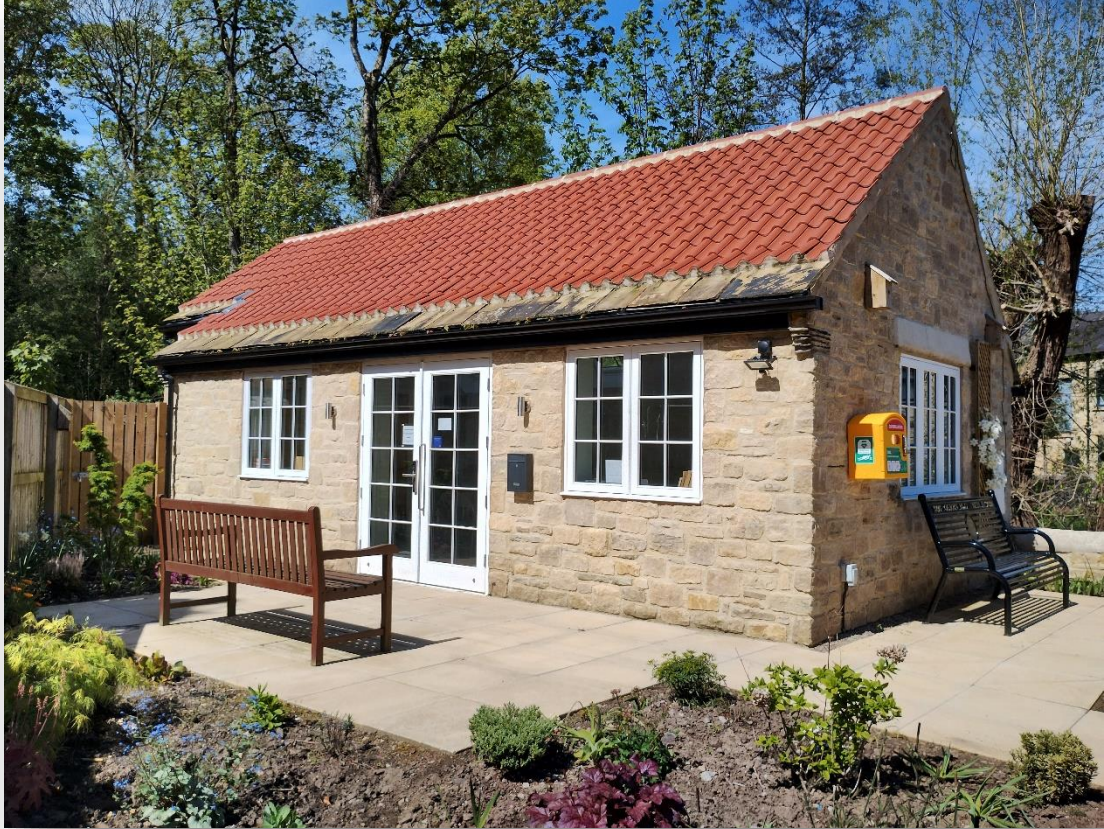
New Bramham Parish Centre
